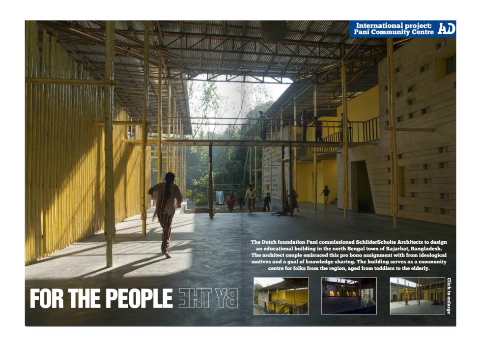
uring the design process attention was mainly focused on locally available materials and weather conditions. The starting point was to realize a building using materials and skills from within a 15 miles radius around the site. Bamboo, hand-shaped brick, Mango wood, reused steel, local mortar and wafer-thin recycled corrugated panels are the main materials used in the building.
